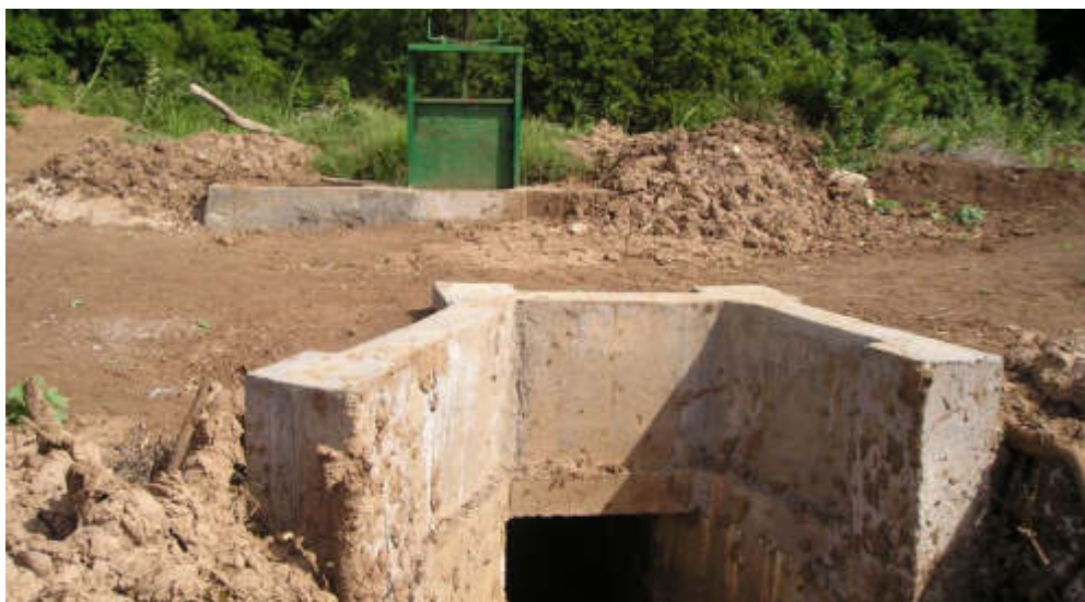
Figure 5.12: Small irrigation channel equipped with a gate
