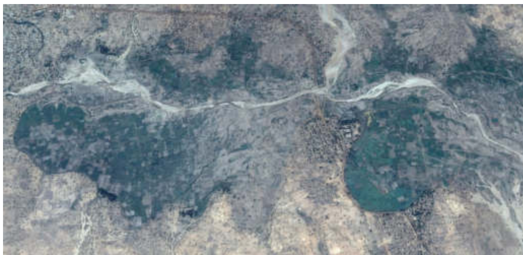
Figure 7.3: Dikes parallel to the river trap part of the flood-wave and rehydrate large alluvial areas (Keita, Niger)
