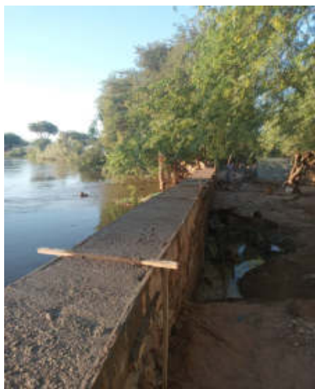
Figure 5.5: Flood retention walls upstream of Beledweyne (constructed by Hiran Development Program in collaboration with community-led initiatives)
