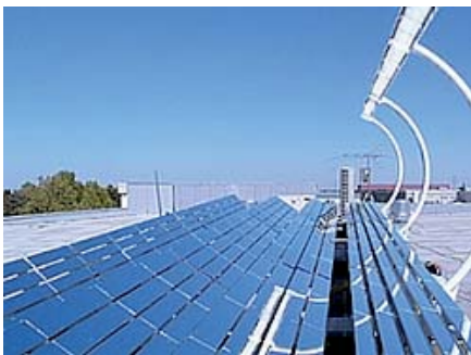
Fig. 3-3. Principle of fresnel reflector systems. BdS 2009.
